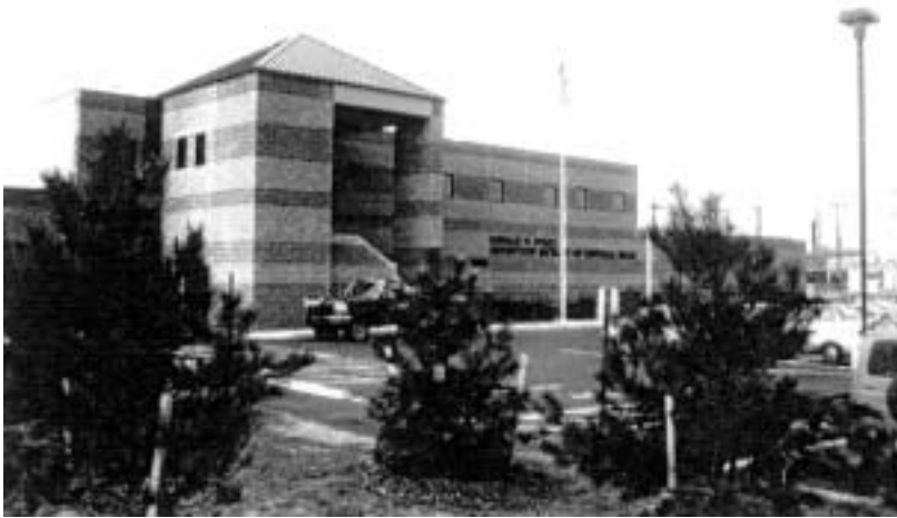
Fig. 3.6: The Donald W. Wyatt Detention Facility (Durrant Group Inc.).
